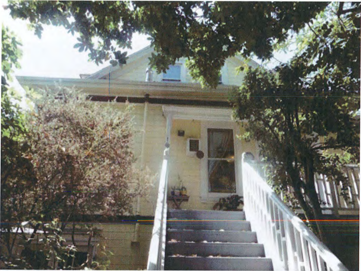
Figure 9: Above, portion of rear elevation showing rear gable, rebuilt staircase from back porch to garden, and double hung windows with casework. Compared to main front facade of the house there is no shingling in the rear gable. Photo 2019.
