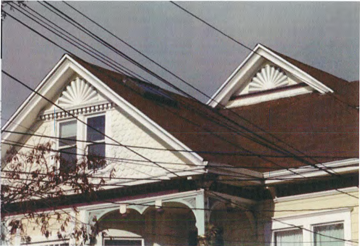
Figure 11: detail view of upper front facade, showing fish-scale shingling, wooden millwork at porch, and wooden sunburst patterns in the gables. Photo 2019.
